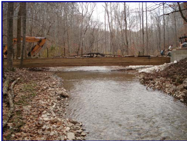
Single Span, 60'-0", Multiple Glu-Lam Timber Girder Trail Bridge
