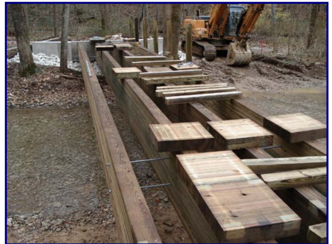
Single Span, 60'-0", Multiple Glu-Lam Timber Girder Trail Bridge
