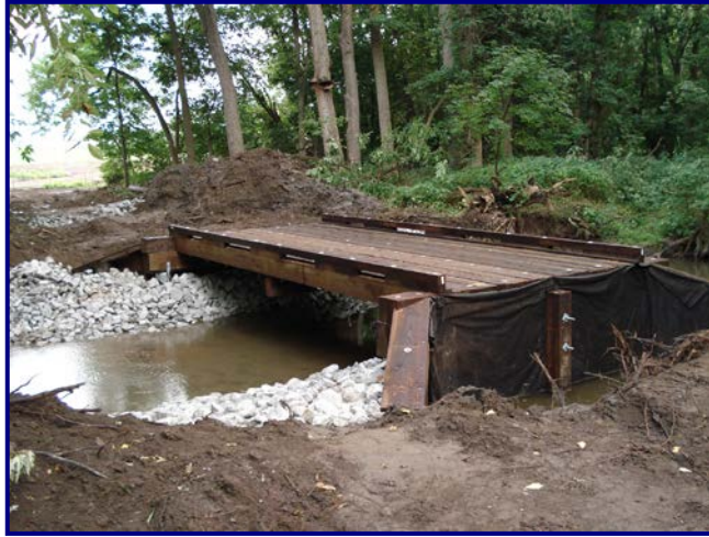
Single Span, 24' Panel Lam Timber Pedestrian Path Bridge
