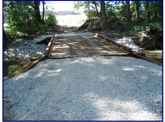
Single Span, 24' Panel Lam Timber Pedestrian Path Bridge
